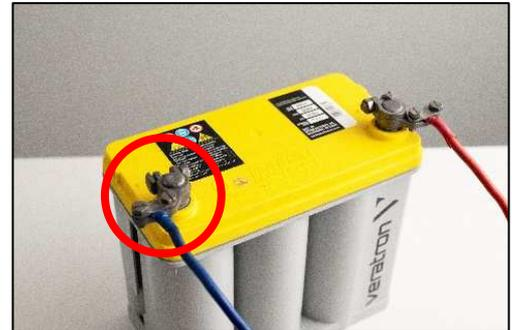
Mount at first the wire harness' ground cable on the IBS ground bolt.
